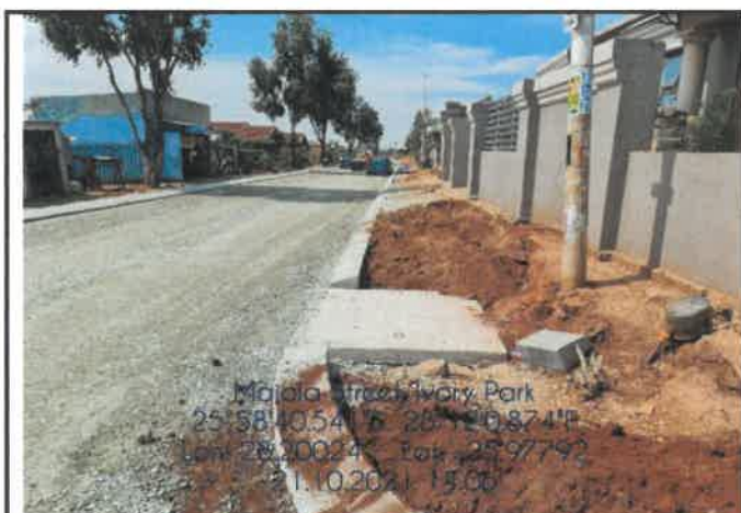
Image 3: Gravel road upgrade-Ivory Park
