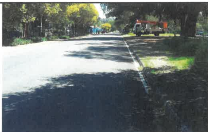
Image 2: Road Resurfaced, Florida, Westlake Road, Region C
