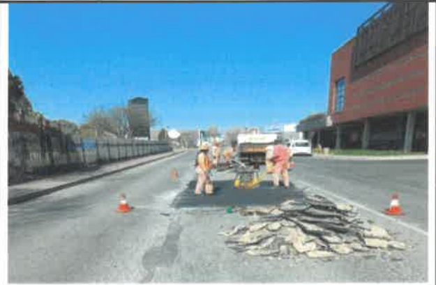
Image 12: Patching, Stone Haven Road, Paulshof, Region A
