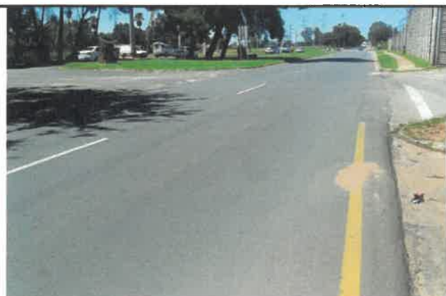
Image 1: Road Resurfaced, Florida, Westlake Road, Region C
