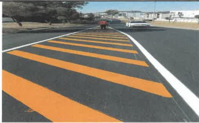
Image 11: Road Markings, Walton Avenue, Midrand
