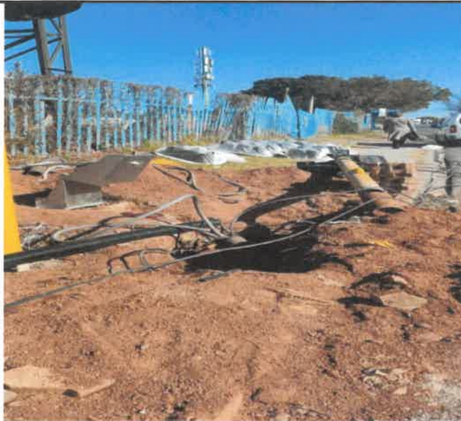
Image 7: Northview Road, Region E-Traffic poles maintenance
