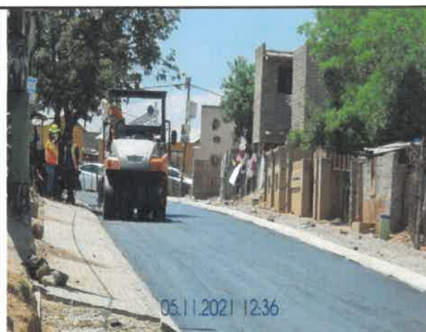
Image 4: Gravel road upgrade- Ivory Park
