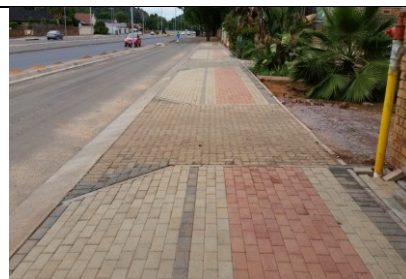
Figure C2.2: Photo no TGSIs required; vehicle access raised to walkway
