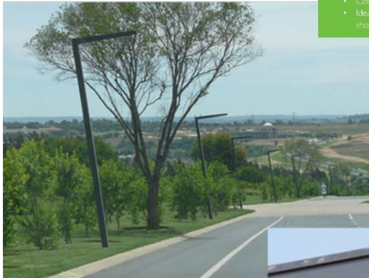
LED street lighting installation Steyn City, Johannesburg
